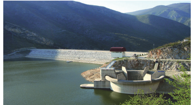
Figure 2. Kozjak Earthfill Dam
