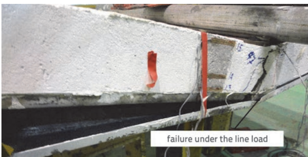
Figure 15. Vertical separations in side of slab
