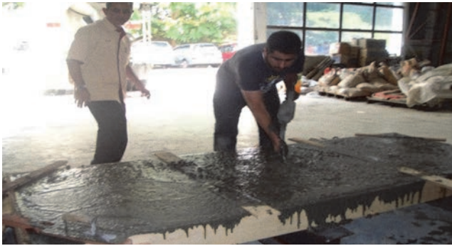
Figure 7. Concrete casting and curing
