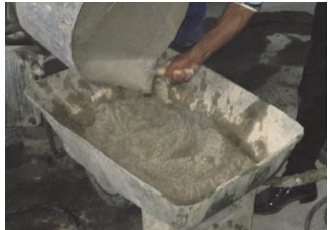
Figure 1. Preparation of traditional Horasan mortar
