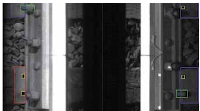
Figure 9. Track surface inspection system – defect detection (missing spikes) [10]
