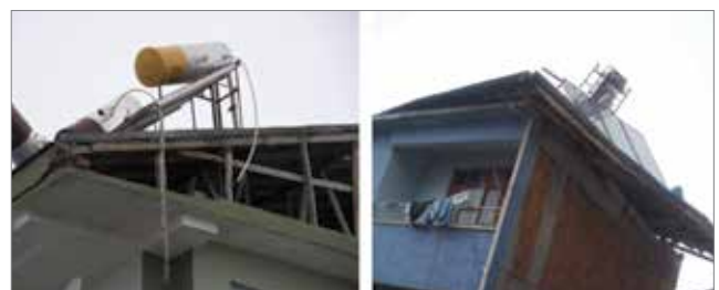
Figure 19. Swayed roofs due to low stiffness and additional seismic masses in Erciř
