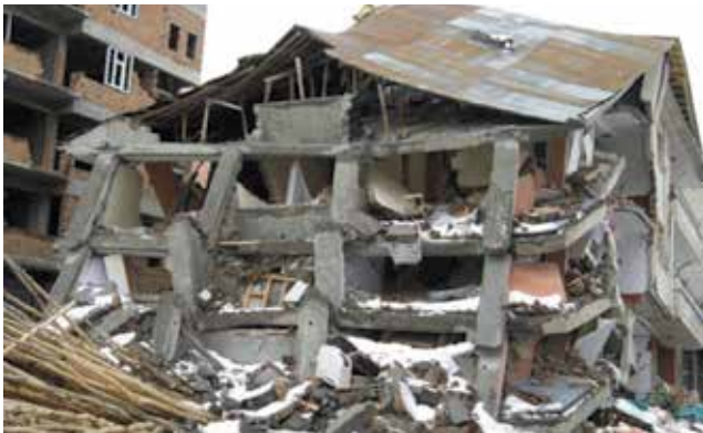
Figure 10. Total collapse of a building in Erciş due to sway mechanism after plastic rotation at the end of each column of individual storeys
