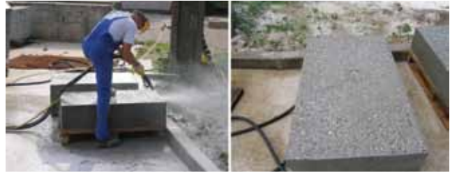
Figure 4. Top concrete surfaces of blocks A and B subjected to water jet treatment with sand (sandblasting)
