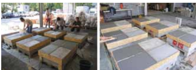
Figure 7. Reshaping concrete freshly placed onto the surface of all 6 blocks
