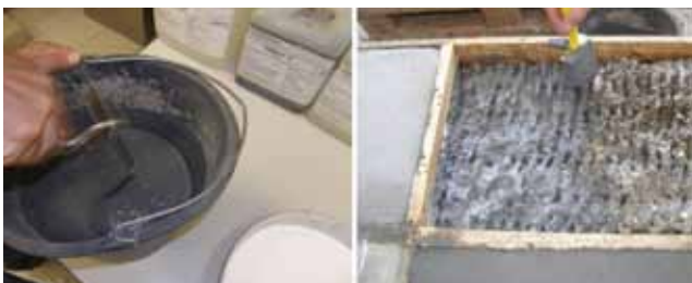
Figure 6. Preparation of binder: proportioning and manual mixing of mortar with latex marked LMC+, and rubbing into the surface of blinding concrete
