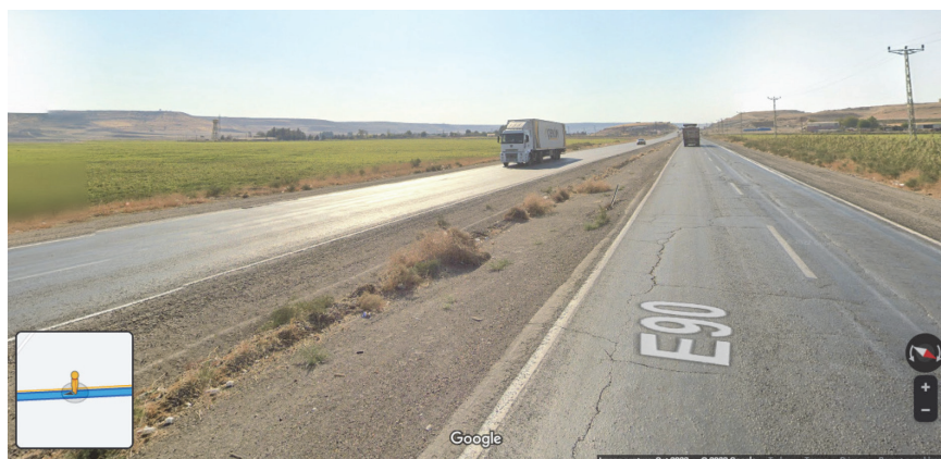
Figure 4. Cizre-Silopi highway platform and pavement view from Google Earth [60]
