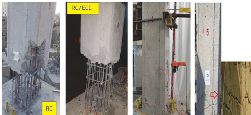
Figure 10. Failure patterns of SP4 (ECC) and SP5 (RC)
