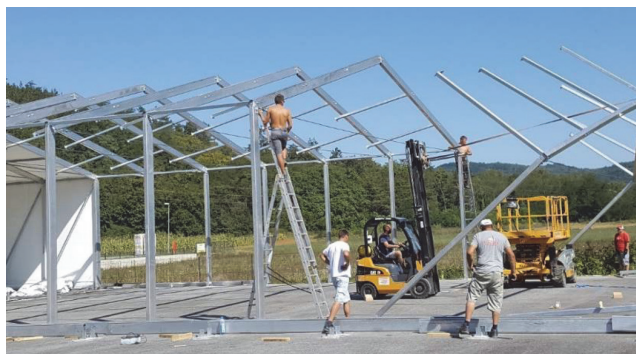
Figure 2. Assembly of aluminium hall
