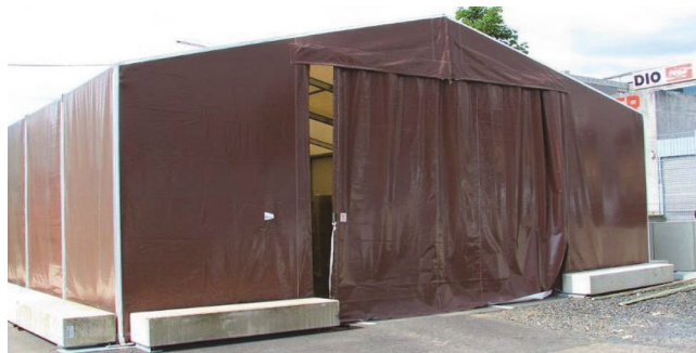
Figure 11. Securing the structure stability through ballasting (heavy anchor blocks)
