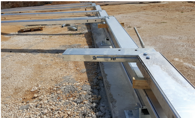
Figure 18. Assembly of frames on the ground
