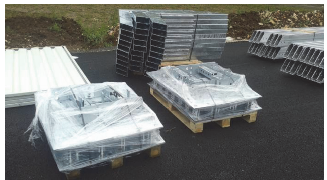
Figure 17. Storage of prefabricated elements at construction site
