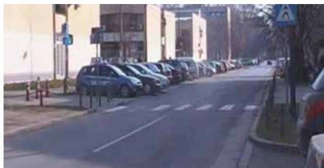
Figure 8. Crosswalk before rehabilitation
