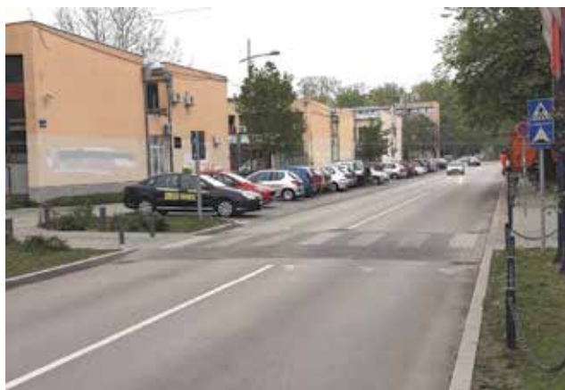
Figure 9. Crosswalk after rehabilitation
