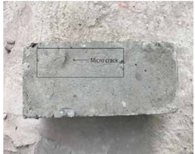
Figure 5. Crack observed in geopolymer bricks at 600 °C after one hour of curing
