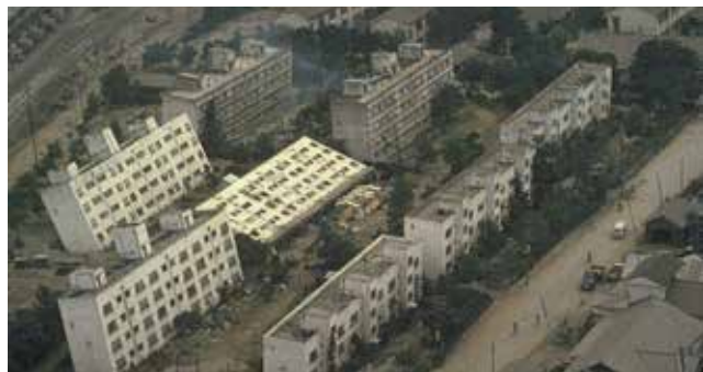
Figure 6. Inclined buildings on liquefied soil in Niigata (Japan) following the 1964 earthquake event, adopted from [18]
