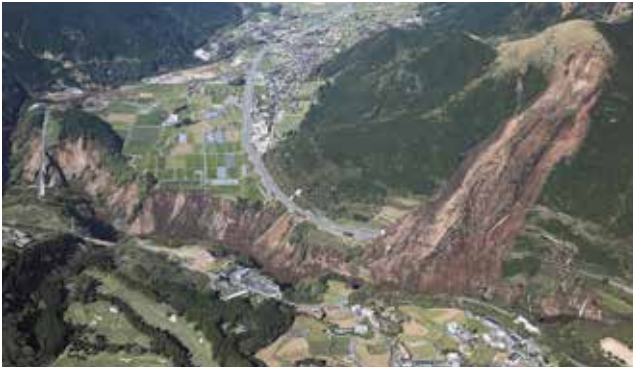
Figure 8. Landslide activated after the magnitude 7.0 earthquake that hit Kumamoto in April 2016, adopted from [25]
