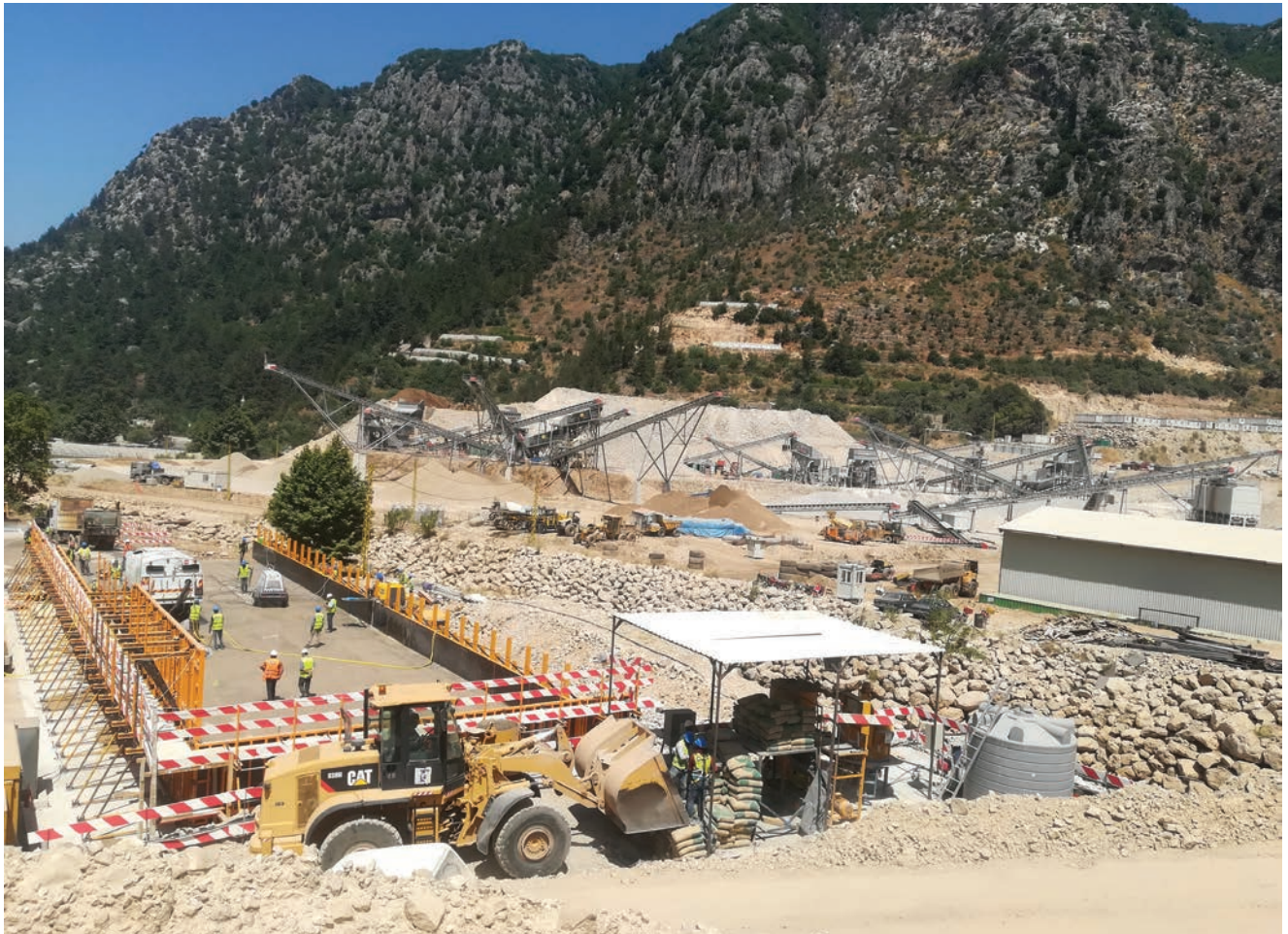
Betoniranje probne ploče (engl. RCC Full Scale Trial Embankment)
