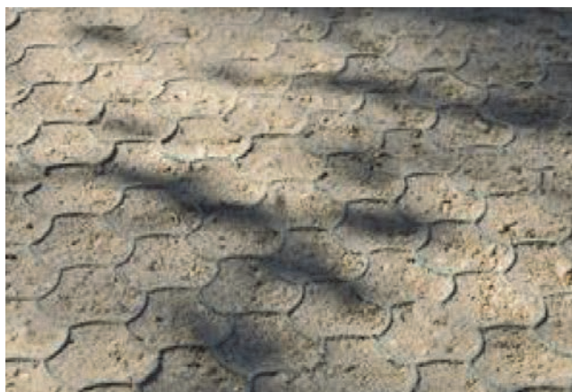
Figure 5. Geocells in pavement structure before asphalt laying
