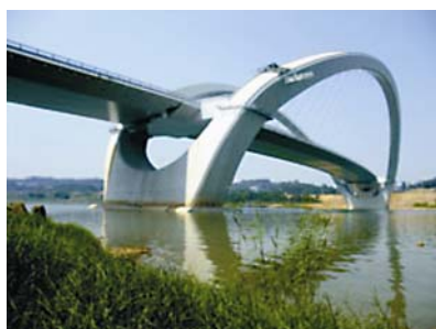
Pogled na most Nanning
